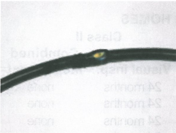
1a Damage to power cable sheath
