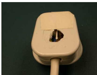
Damage to mains plug.
