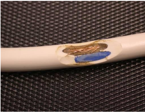
Damage to power cable sheath.
